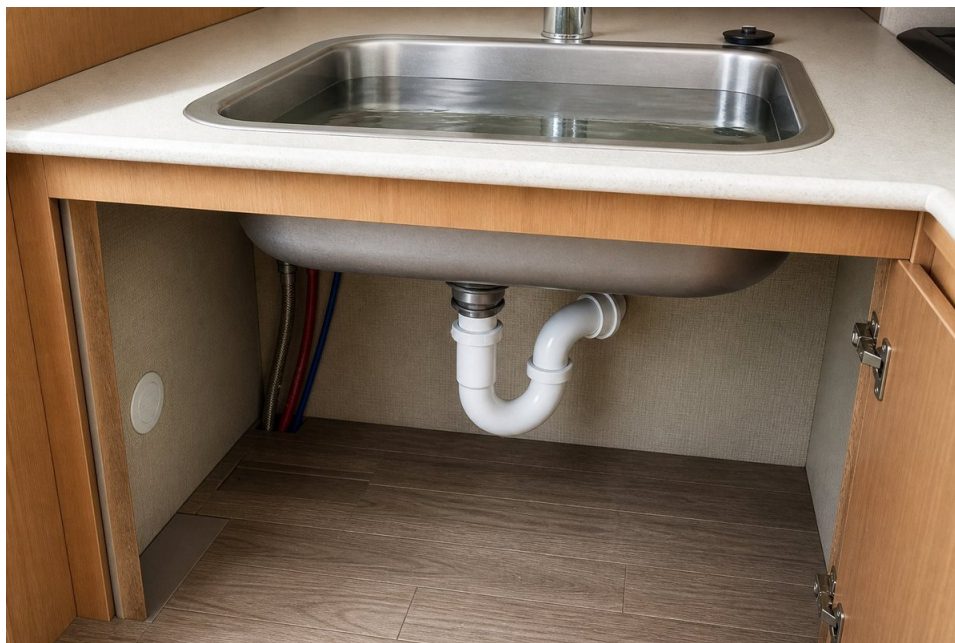
Illustration: Sink drain and accessible under-sink plumbing
