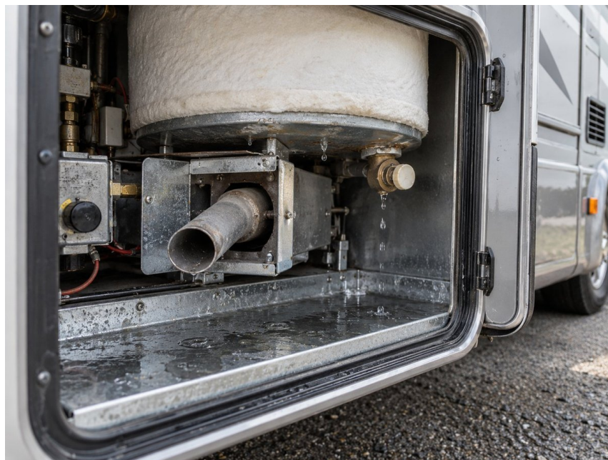
Illustration: Water-heater service area and visible water accumulation.
