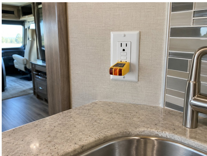
Illustration: Kitchen receptacle and GFCI test setup; the functional result is described above.
