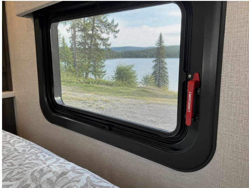
Illustration: Bedroom emergency exit window and release hardware; opening failure is described above.
